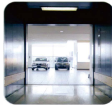
∞ Front-and-rear opening elevator car
